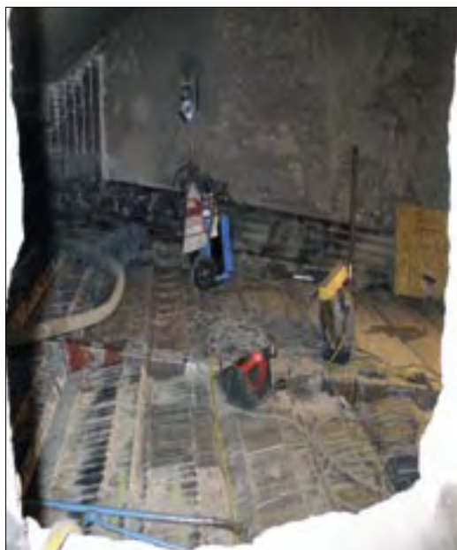
Figure 9. A stoker-fired boiler during cleaning. The grates in the base of the boiler transport the fuel during combustion.
