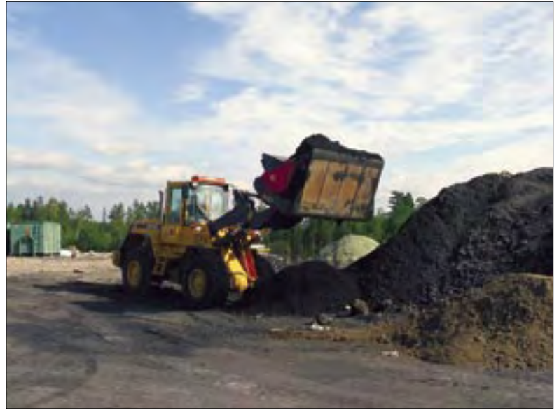
Figure 13. Crushing with a sieving bucket, a tractor-mounted bucket with rotating crushing cylinders fitted in the base.
