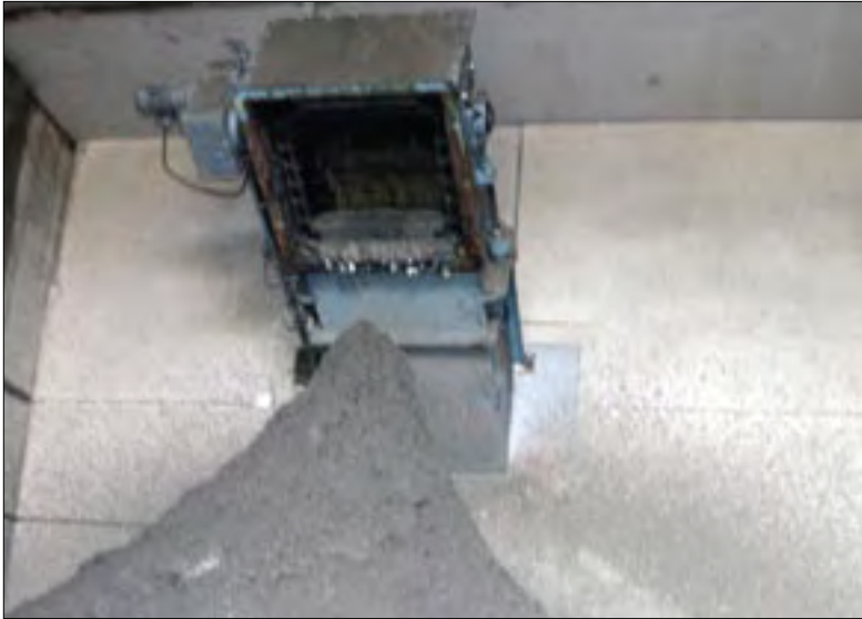
Figure 10. Wet outfeed ash at Sannaverket in Kristinehamn, Sweden.
