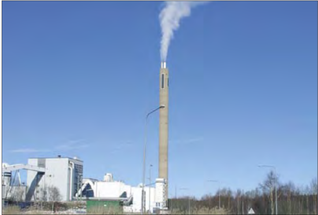
Figure 7. Heden, a district heating plant in Karlstad, Sweden, which uses pure forest fuel.
